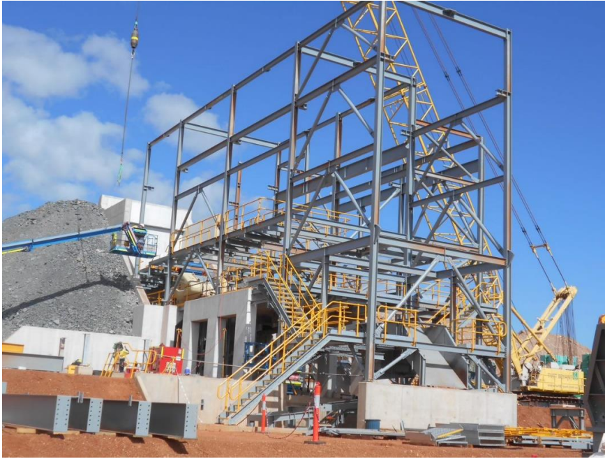
Figure 6 – Crushing area steelwork (Photo taken 11 June 2022).
