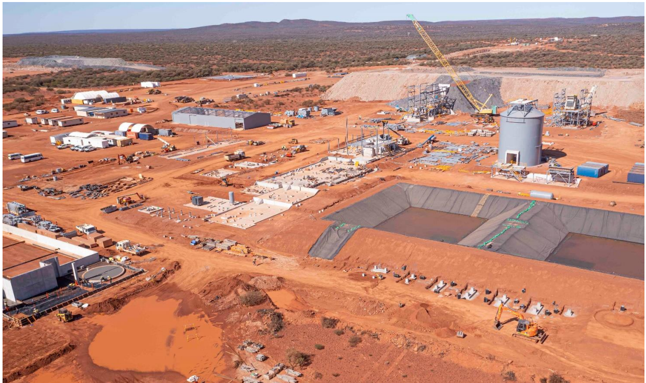
Figure 5 – Processing plant construction (Photo taken 7 June 2022).
