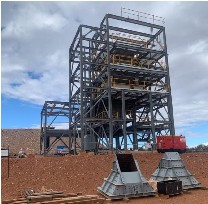
Figure 7 – Screening area steelwork (Photo taken 12 June 2022).
