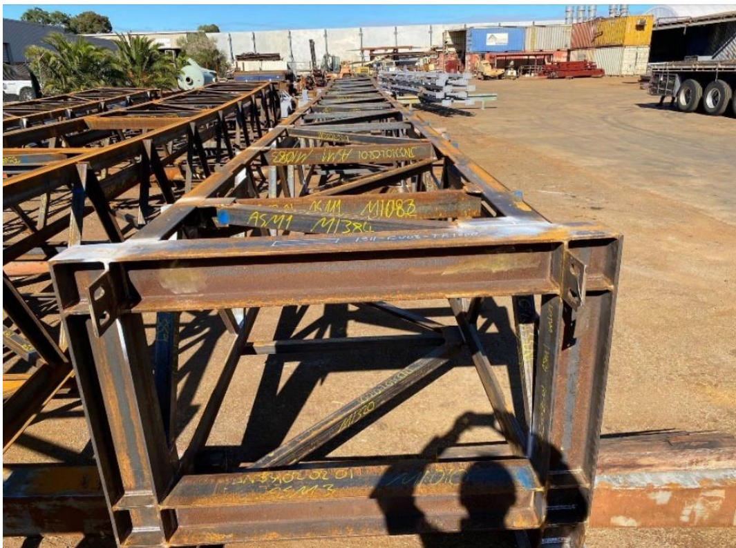
Figure 9 – Conveyor truss fabrication in Perth.
