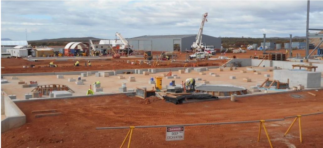
Figure 8 – Flotation area concrete work.
