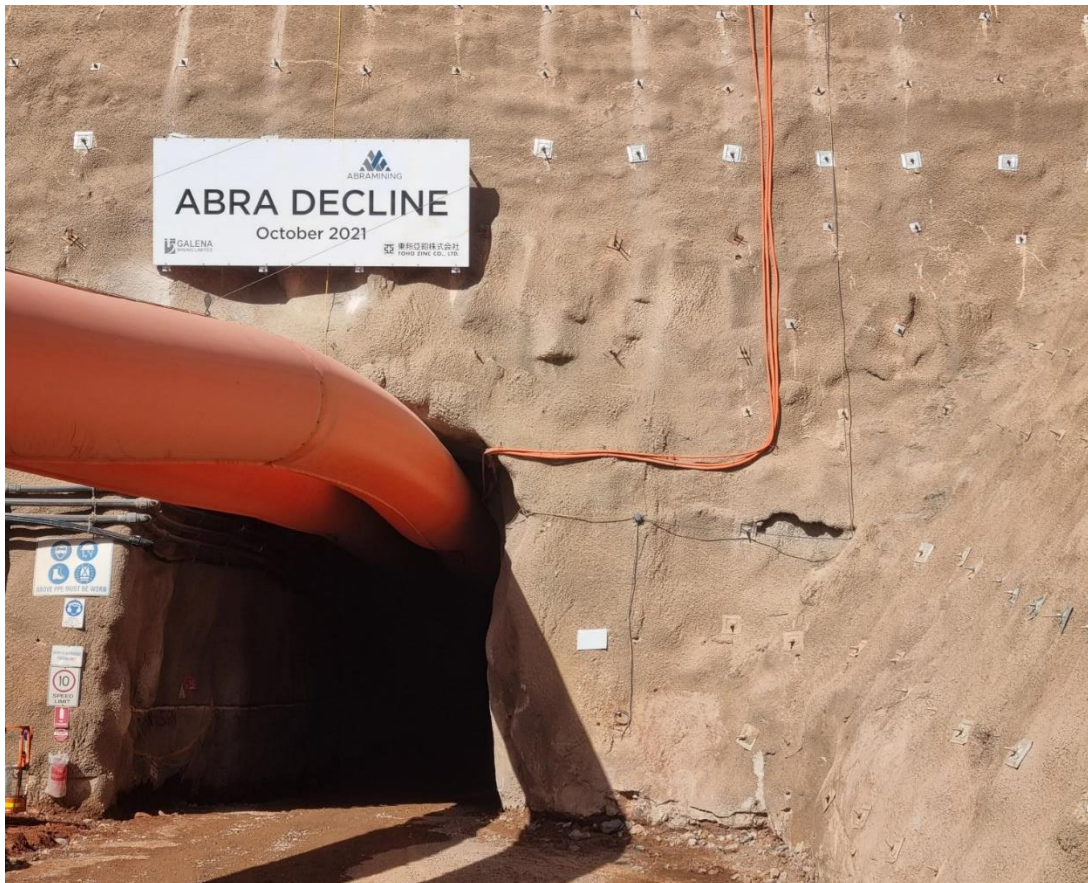
Figure 13 – Abra underground portal.
