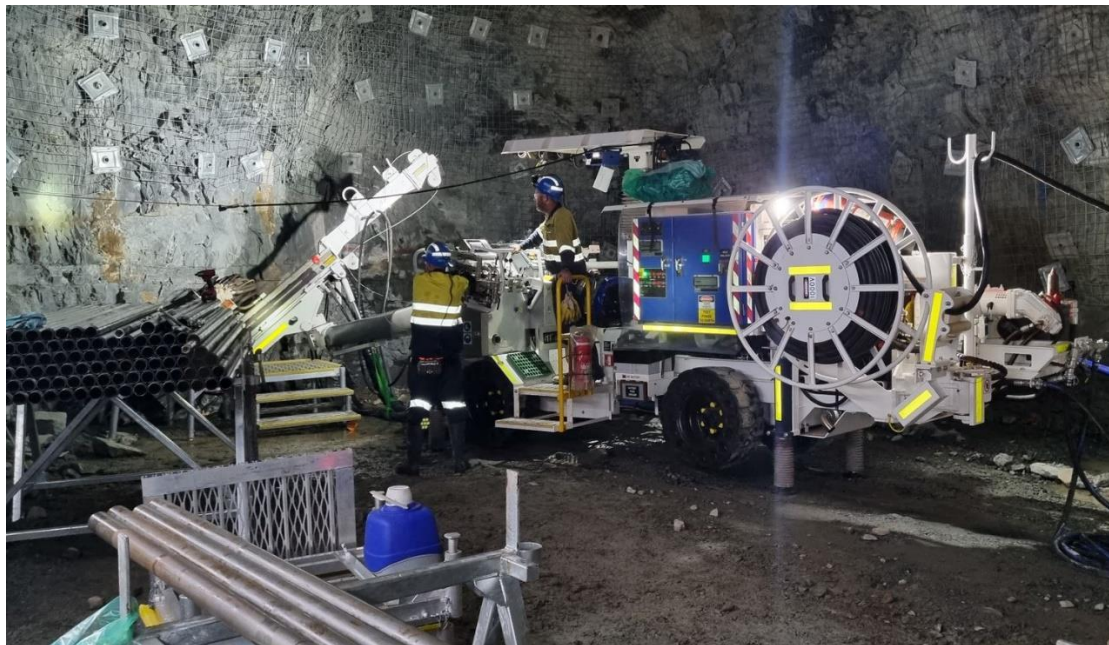
Figure 1 – Commencement of Underground Drilling at Abra (Swick Mining Services).
