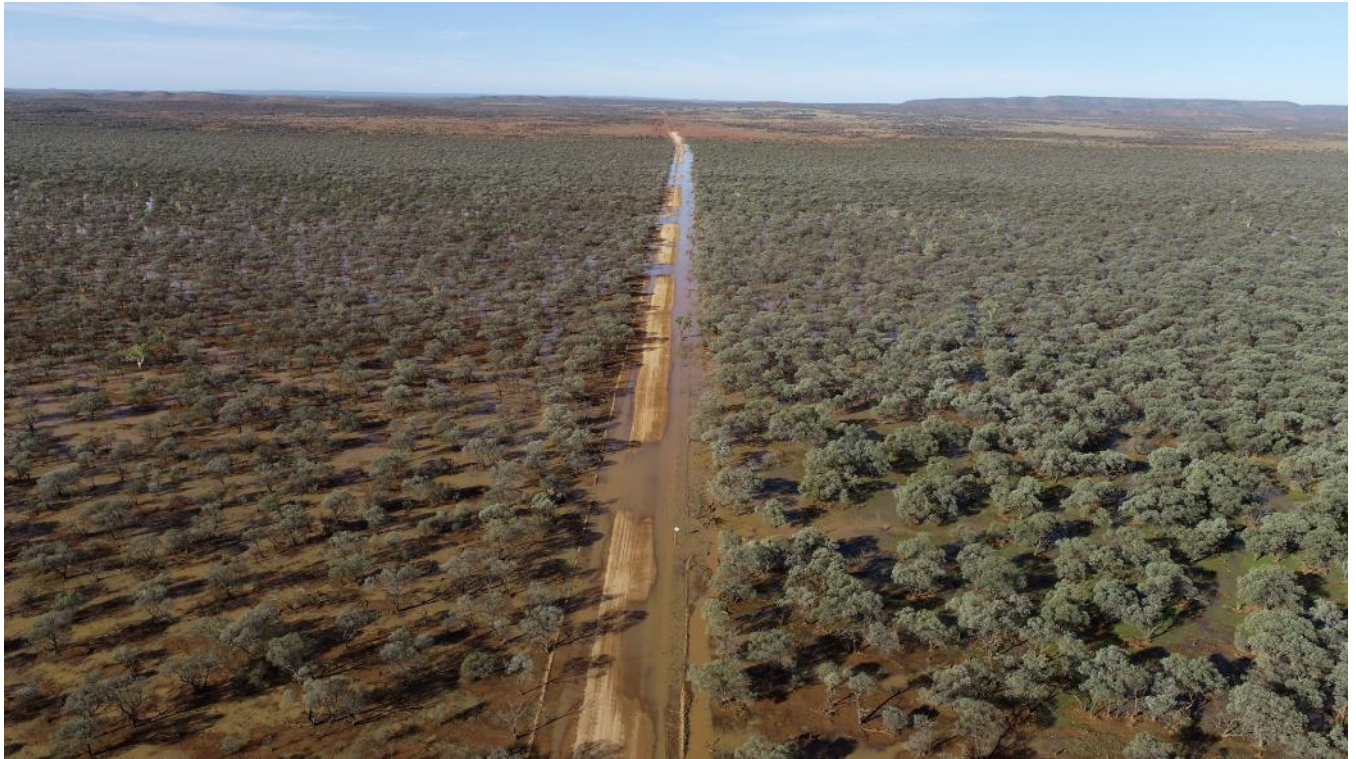
Figure 8 – Ashburton Downs Road, Gascoyne River Crossing (Photo 14 April 2023).
