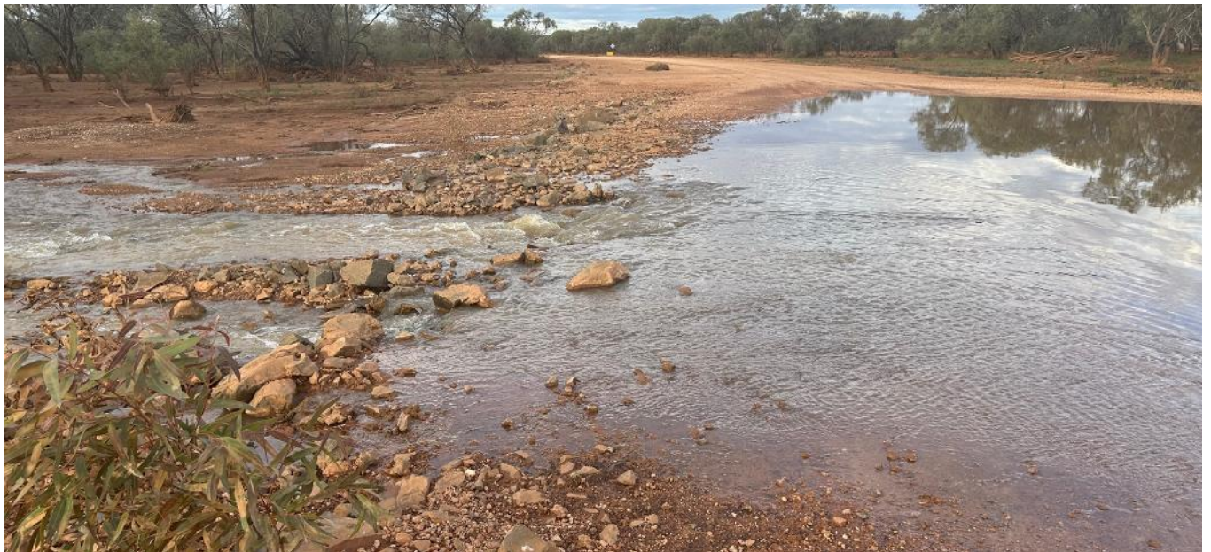
Figure 9. – Ashburton Downs Road, Gascoyne River Crossing (Photo 24 April 2023).
