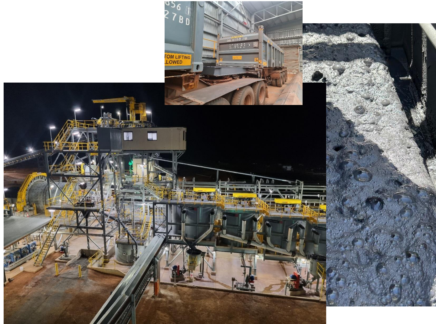
Figures 8, 9 & 10: Abra processing plant, concentrate containers and flotation cell
