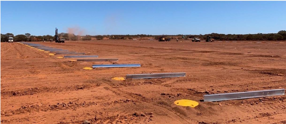
**Figure 7. Post-hole drilling and solar panel supports.**
