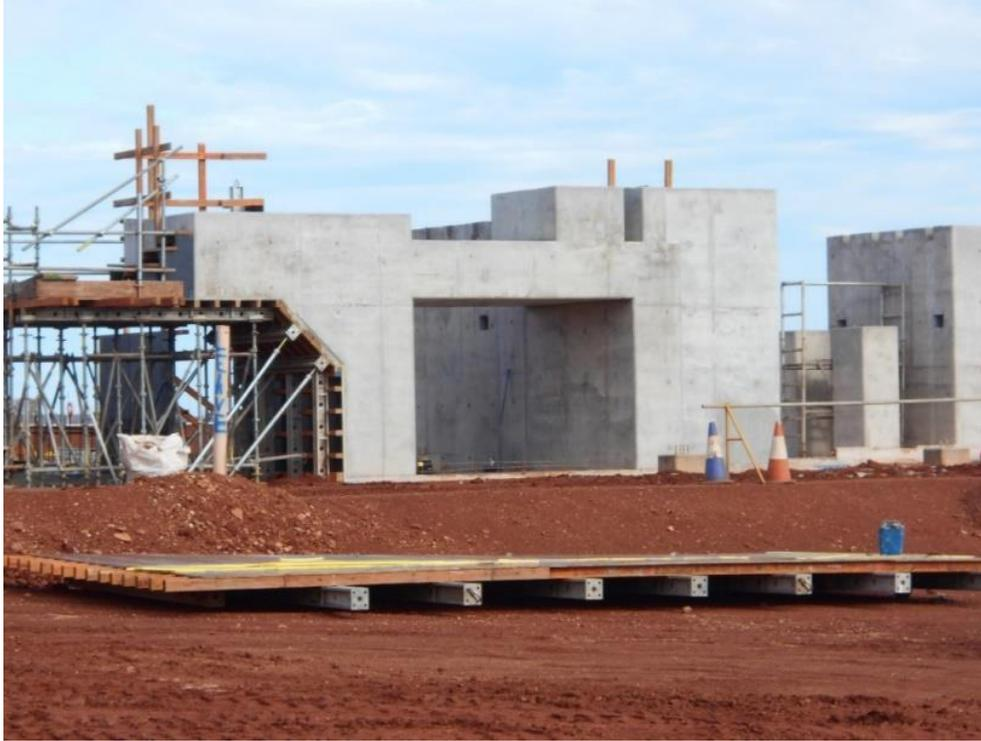
**Figure 6. Grinding mill plinths.**
