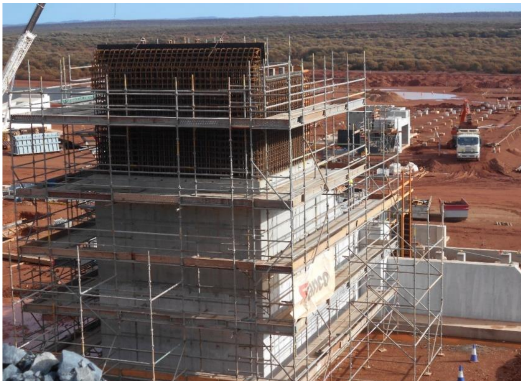
Figure 4 – Crusher concrete and 3rd lift rebar steelwork installed.
