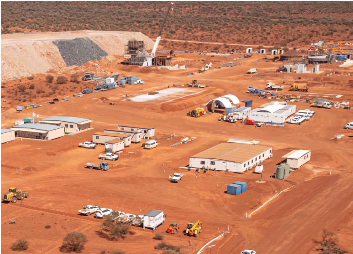
Figure 1 – Work progress at the Abra construction site.
