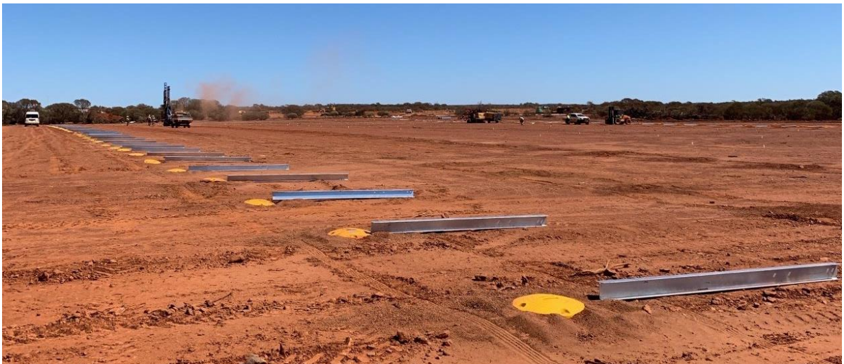
Figure 13 – Post hole drilling commencement for solar panels at Abra.
