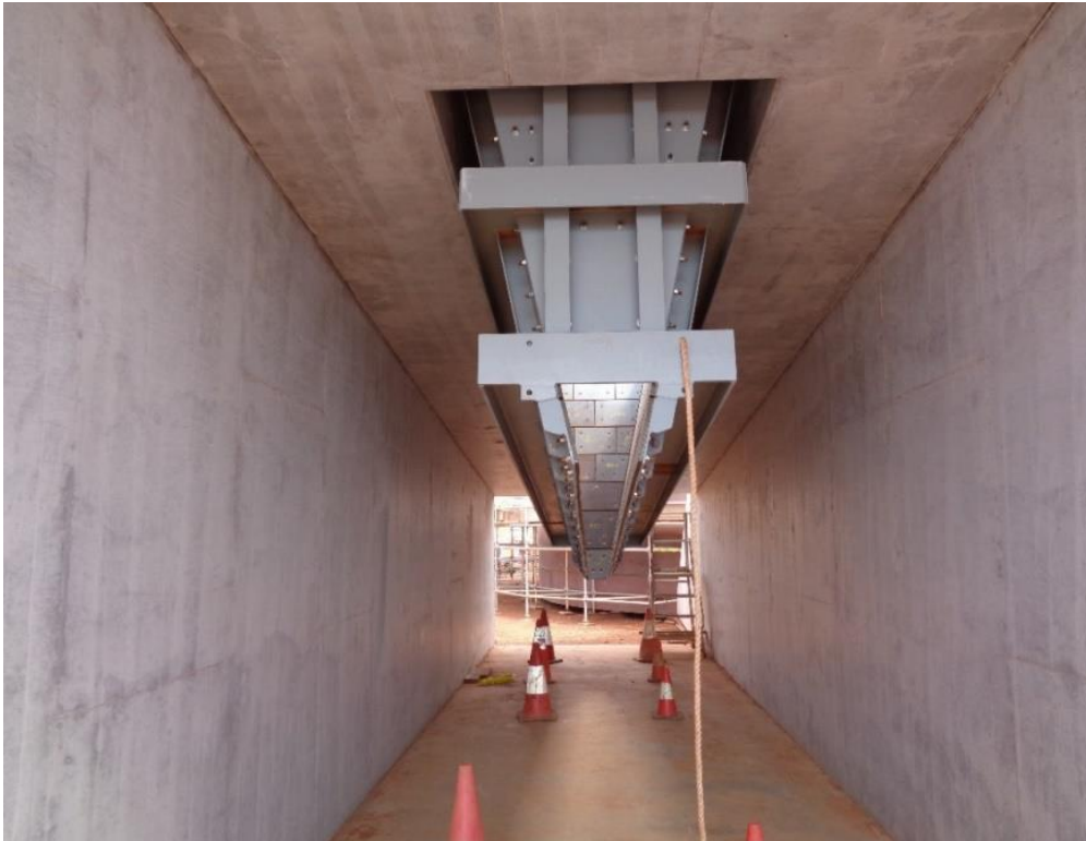
Figure 5 – Fine Ore Bin (FOB) reclaim chute.
