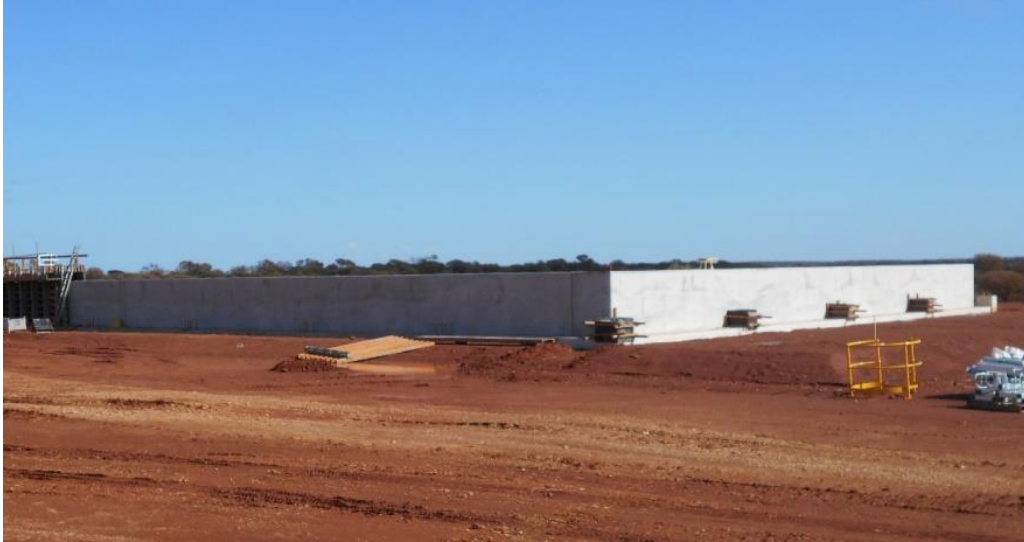
Figure 7 – Concentrate storage shed walls.
