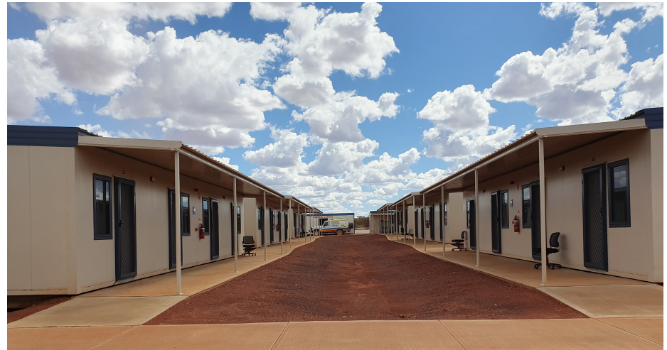
Stage 1 of commissioned permanent camp
