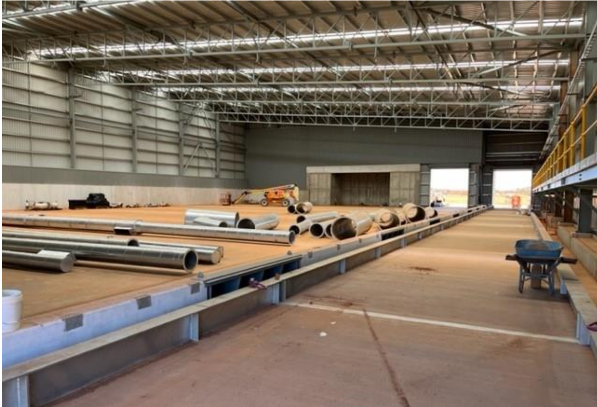
Figure 11 – Inside of concentrate storage shed (Photo 11 November).
