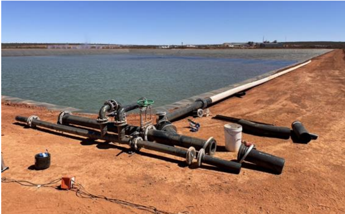
Figure 15 – TSF piping installation.
