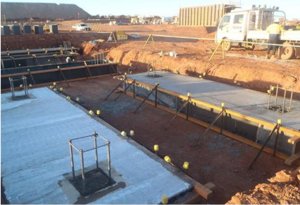
**Figure 5** – Flotation area concrete footings.
