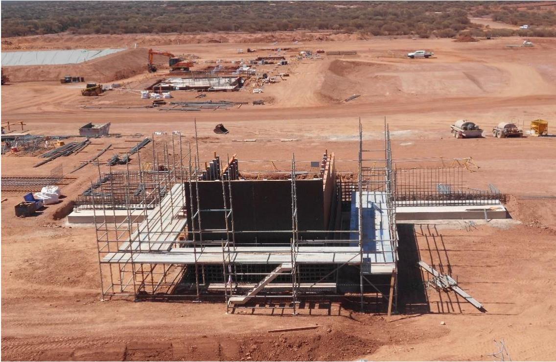
**Figure 3** – Crusher wall formwork in the foreground and the mill concrete foundations in the background.
