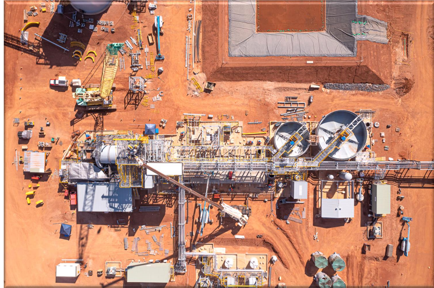
Processing Plant Construction - (Photo September 2022)
