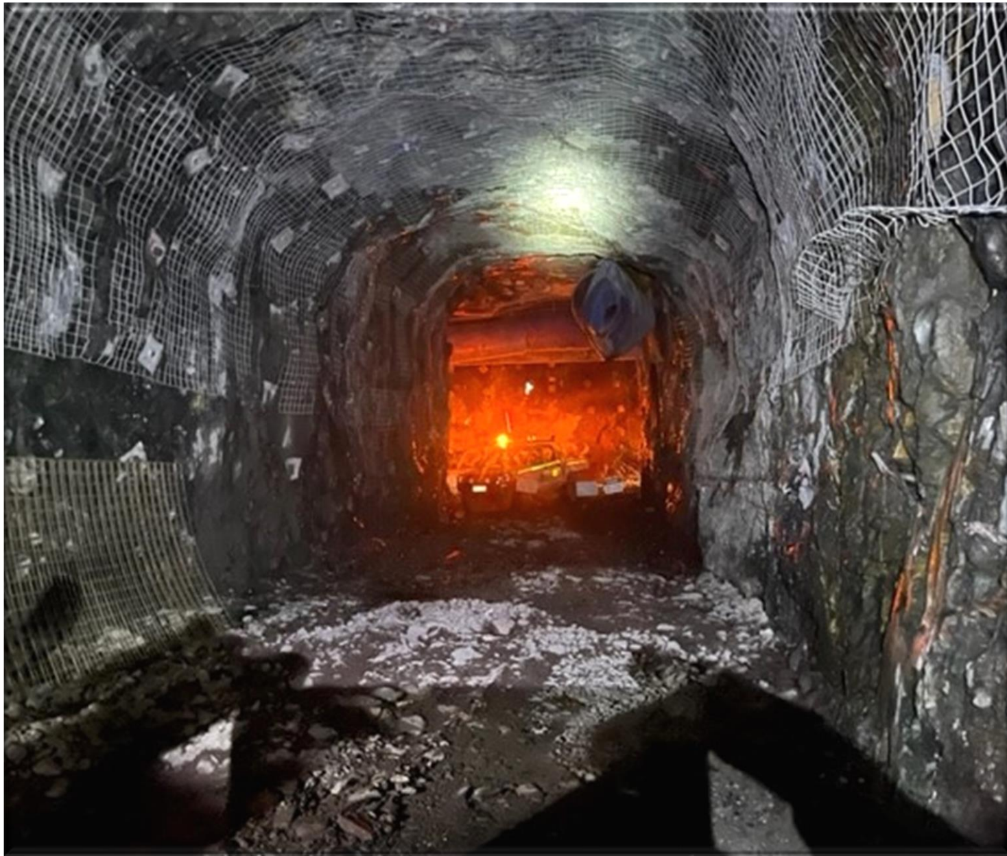
1300 Ore Access Drive
