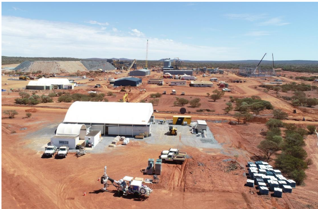
Figure 5 – Abra surface infrastructure showing core processing (foreground), mining workshops (left side), change-house (dark building), offices, and processing facility (background).
