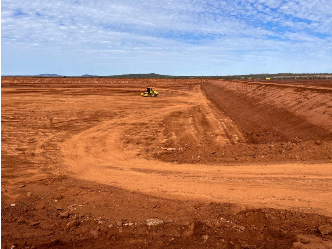
Figure 6 – Abra TFS construction with preparation for liner installation (photo 9 September).
