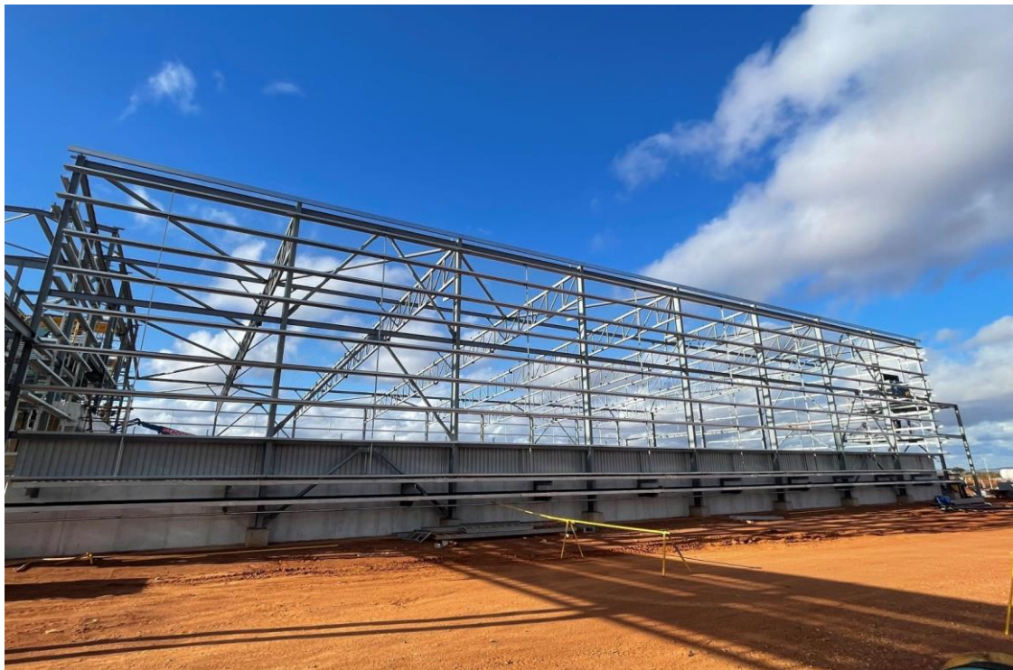
Figure 11 – Concentrate shed construction.
