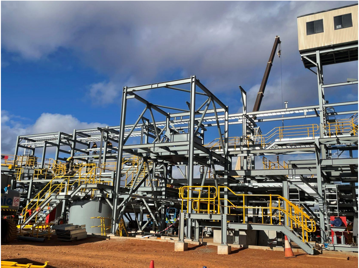
Figure 12 – Flotation section waiting arrival of flotation cells (photo 9 September).
