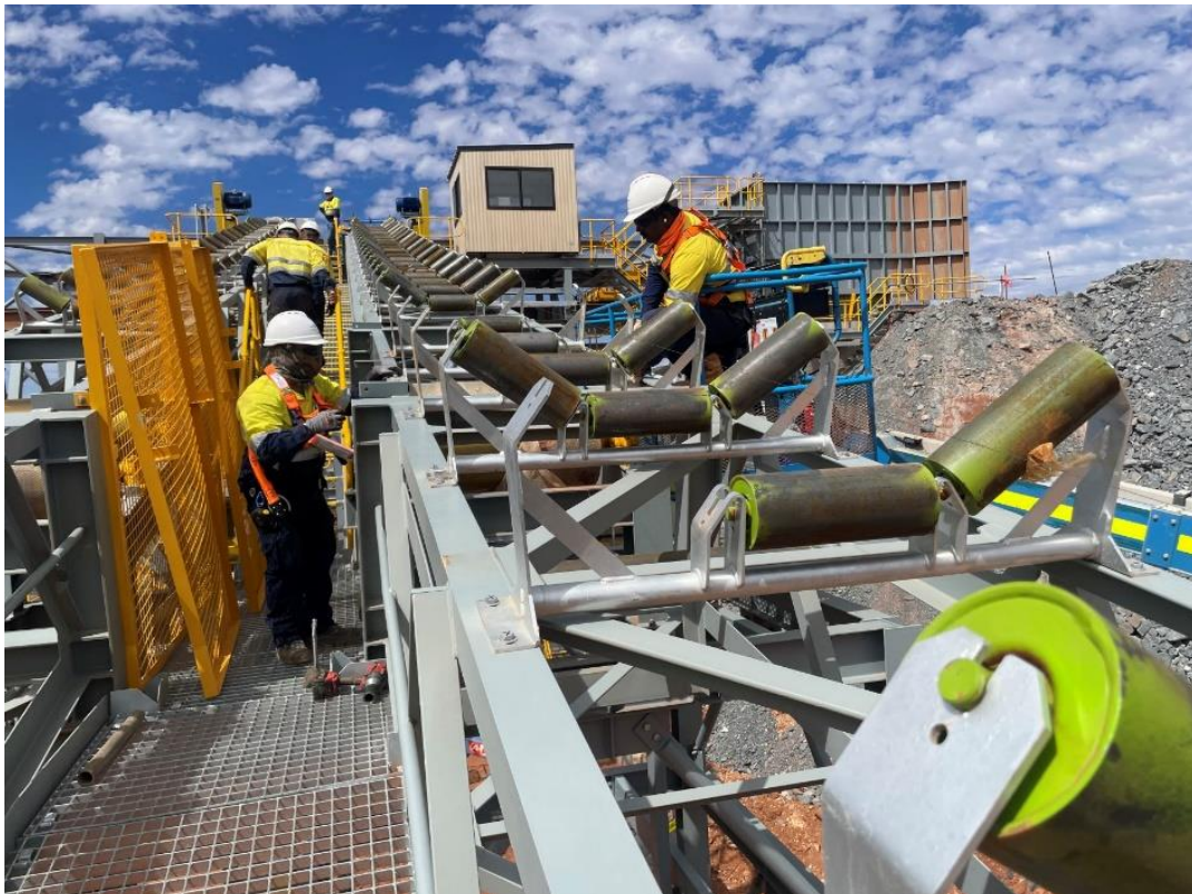
Figure 7 – Abra crushing section conveyor alignment work.
