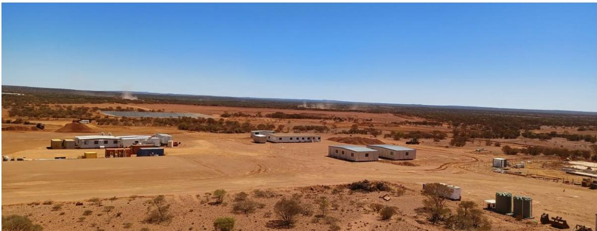
**Figure 3** – Construction offices and mine administration buildings in place. Completed plant site earthworks in the foreground and storm water event pond in the background.
