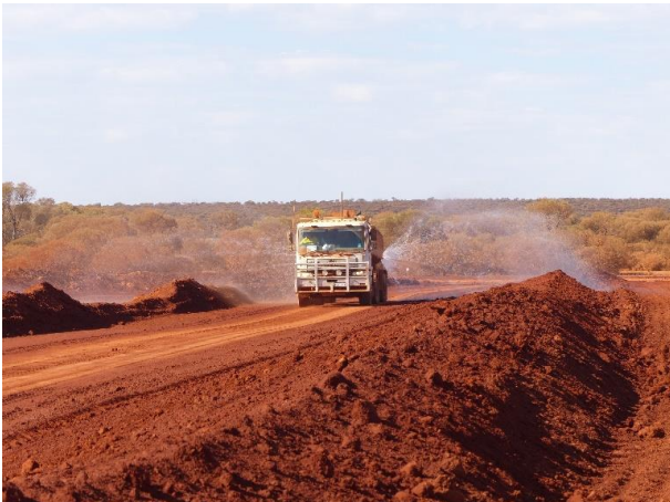
Maintaining OMC on the fill material
