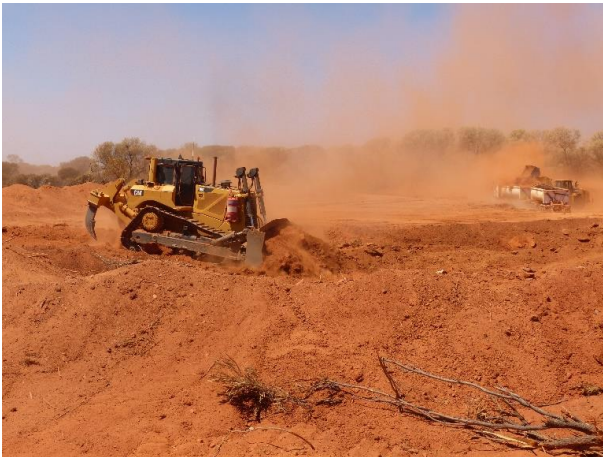
Dozer pushing up fill material
