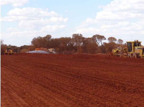
Maintaining OMC on the fill material
