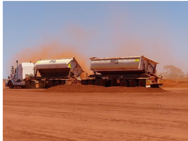
Fill material being placed in the fill
