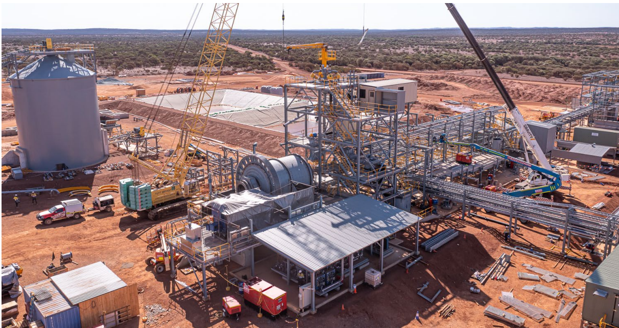
Figure 1 shows the Abra processing plant construction progress (photo: 19 September 2022)
