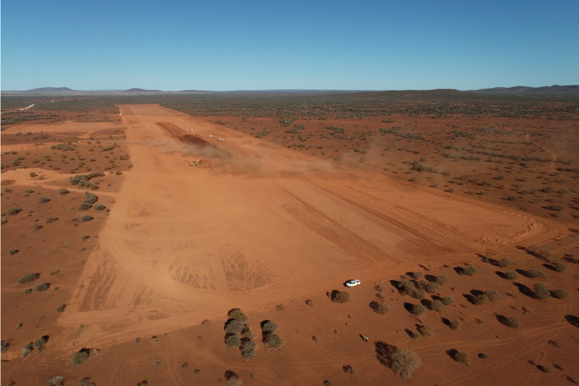
Figure 4 – RDH civil works associated with Abra airstrip construction (September 2021)
