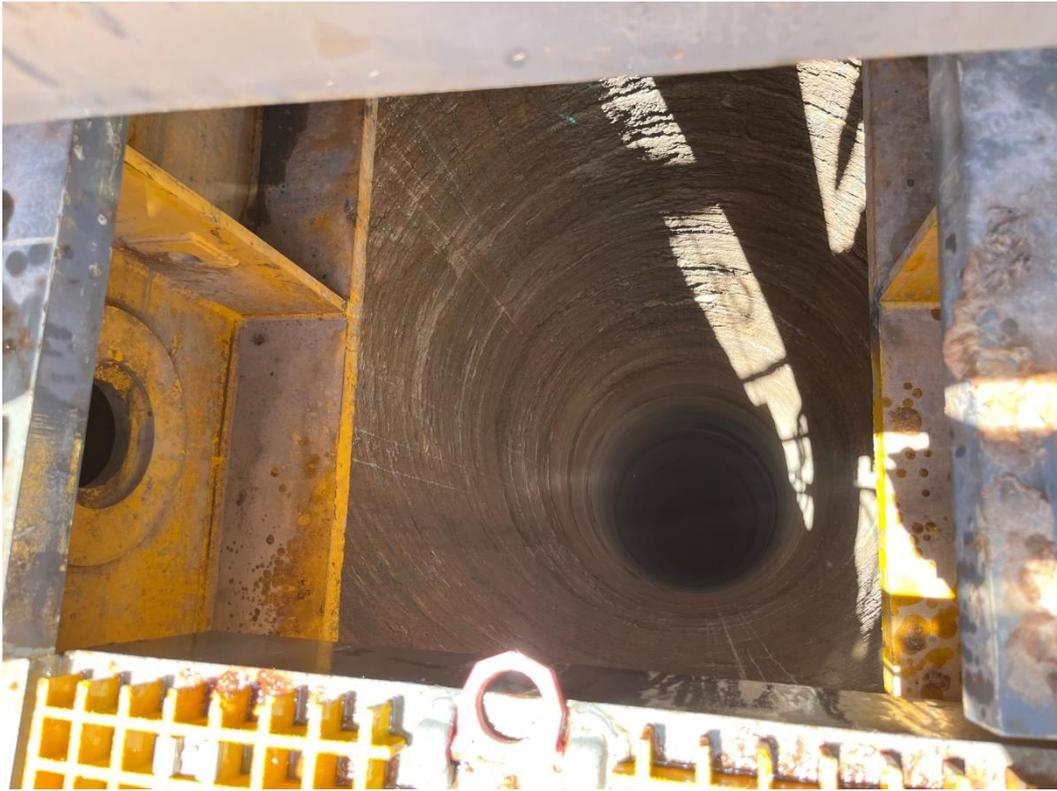
**Figure 13** – Drilling complete of first 4.5m diameter primary ventilation hole looking down from the surface.
