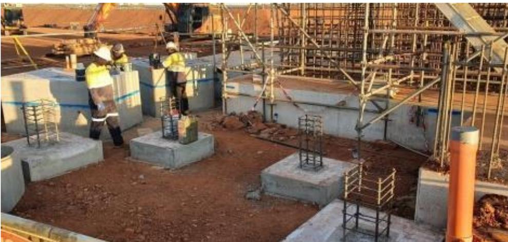
**Figure 6** – Mill area foundations.
