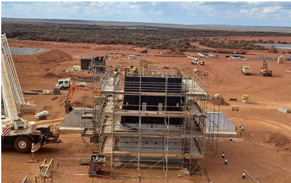
**Figure 3** – February progress on crusher concrete and 2<sup>nd</sup> lift formwork in the foreground and the mill concrete formwork in the background.
