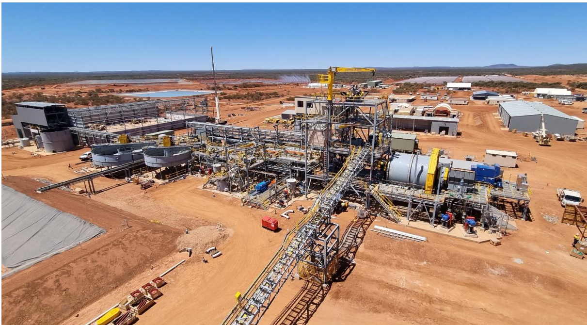
Figure 8. Processing plant showing, milling, flotation, and concentrate sections (Photo – 14 October 2022).
