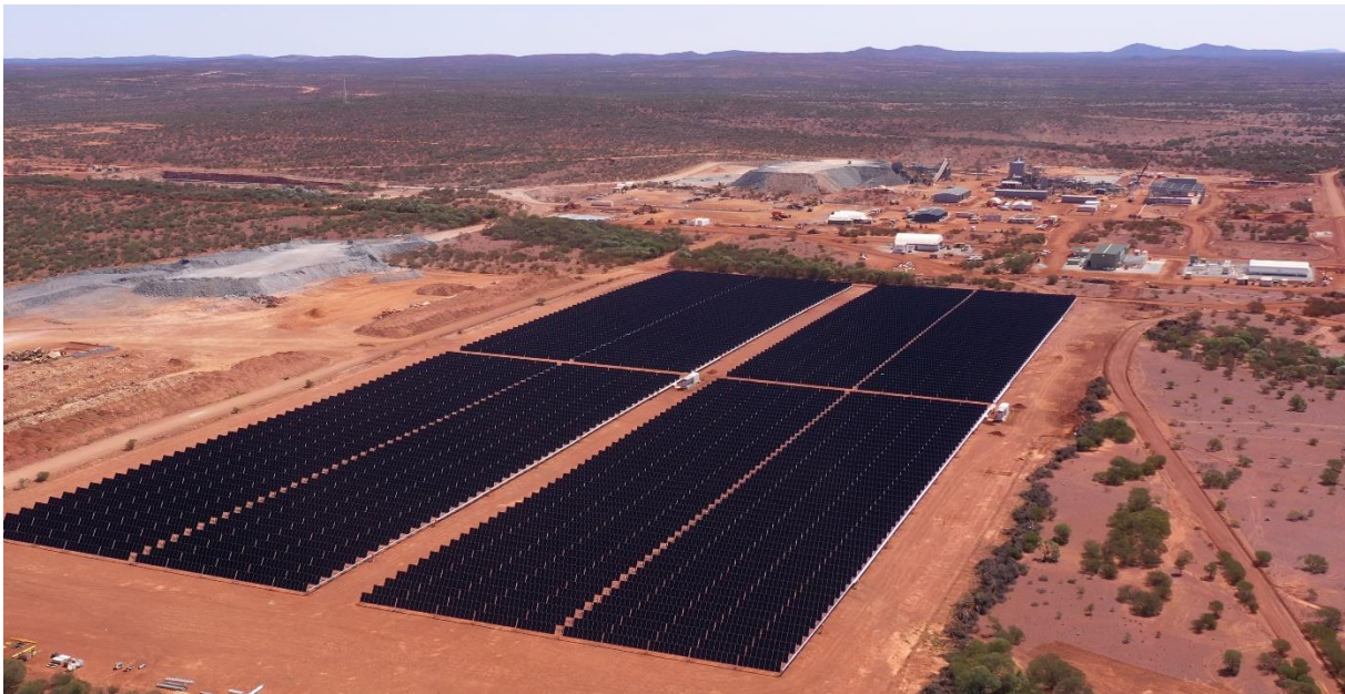
Figure 10. 16,000 solar panels installed in solar farm, ready for commissioning in October.
