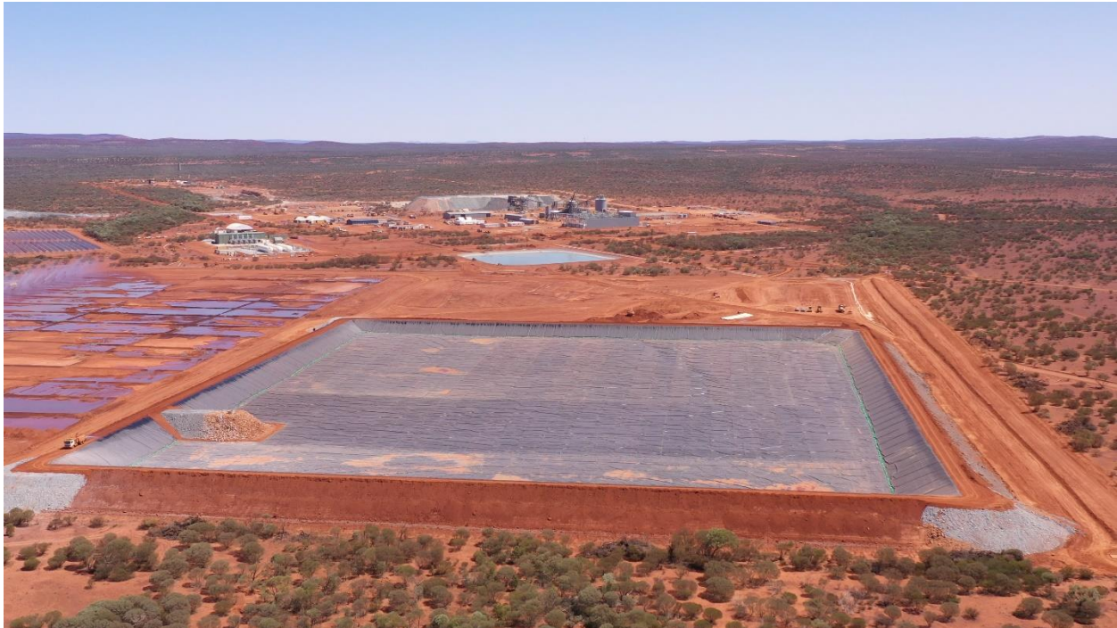
Figure 7. Completed TSF (stage 1) with Abra plant in background and showing mine dewatering evaporation (Photo – 14 October 2022).
