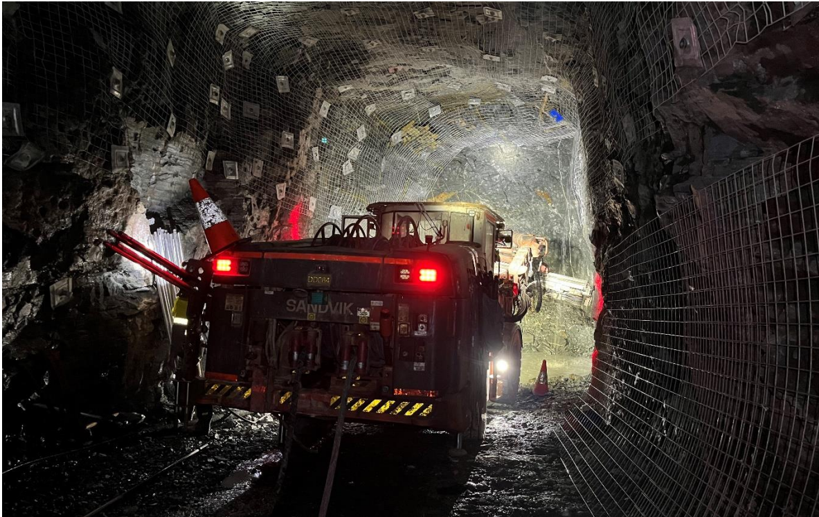
Figure 11. Abra underground decline development (Photo 30 September 2022).
