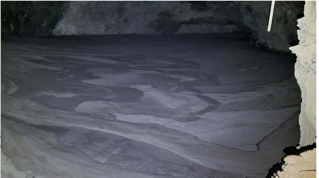
Figure 4 – Abra 1280 level underground cement paste-filling (Photo 27 January).
