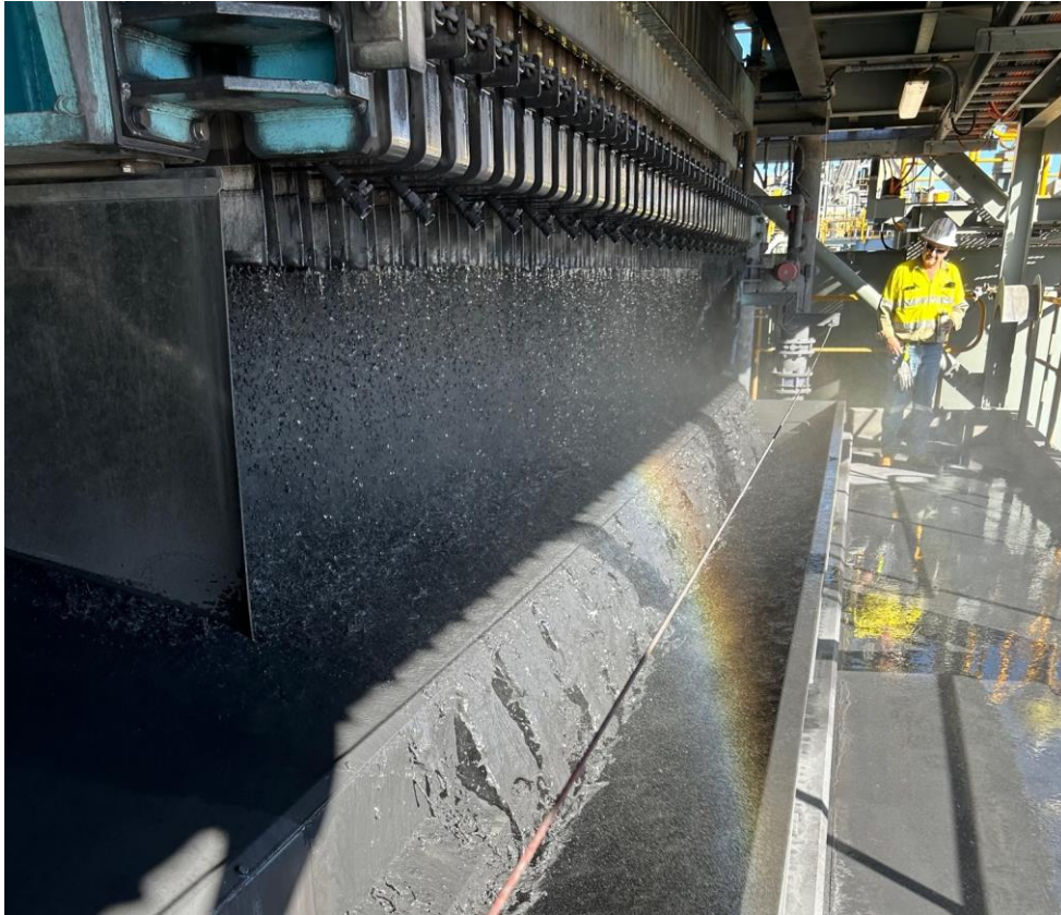
Figure 2 – Ishikawa filter going through cleaning cycle at Abra processing plant (photo 16 May)
