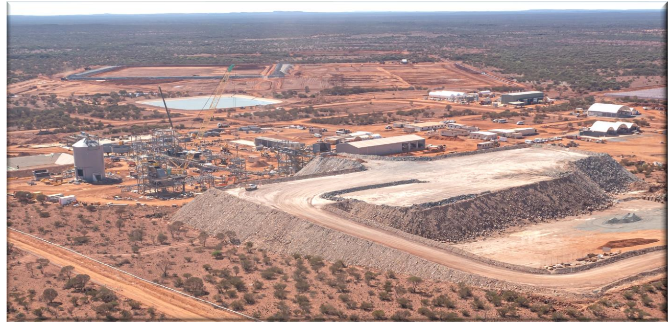
Processing Plant & TSF Construction - July 2022
