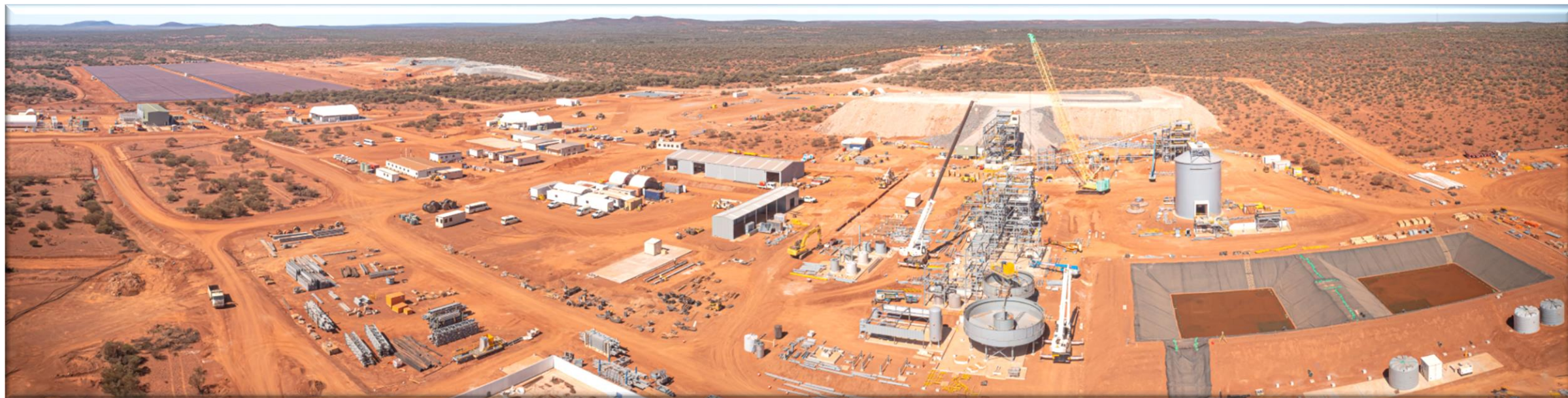
Surface Infrastructure, July 2022
