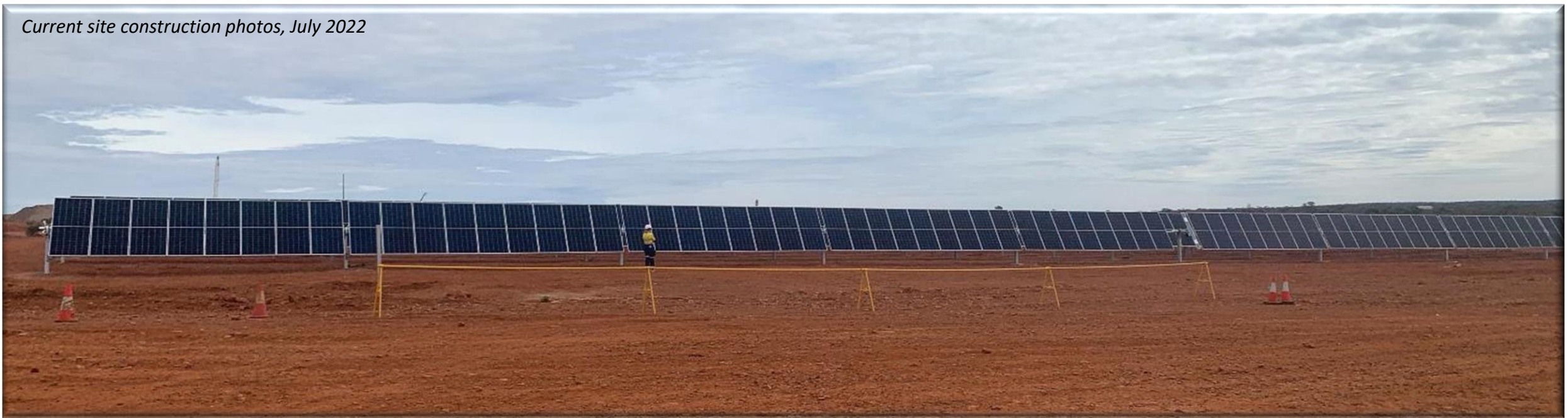
16,000 solar panels installed
