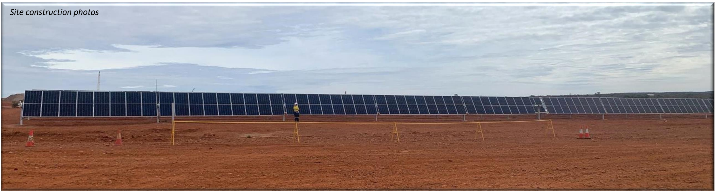
16,000 solar panels installed
