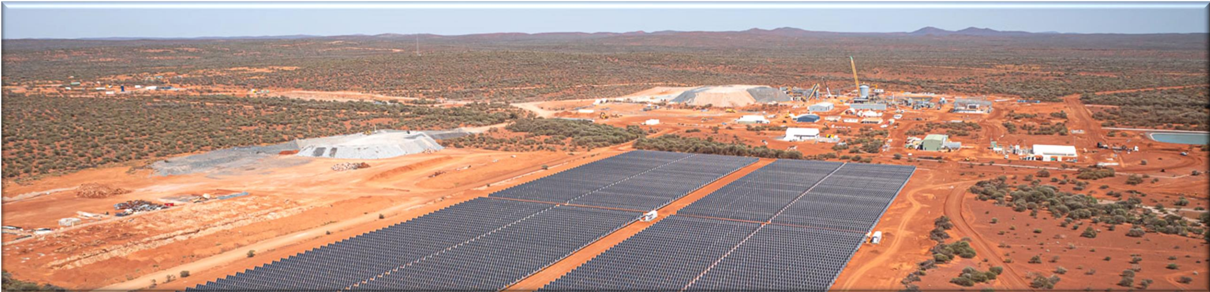
Surface infrastructure, September 2022
