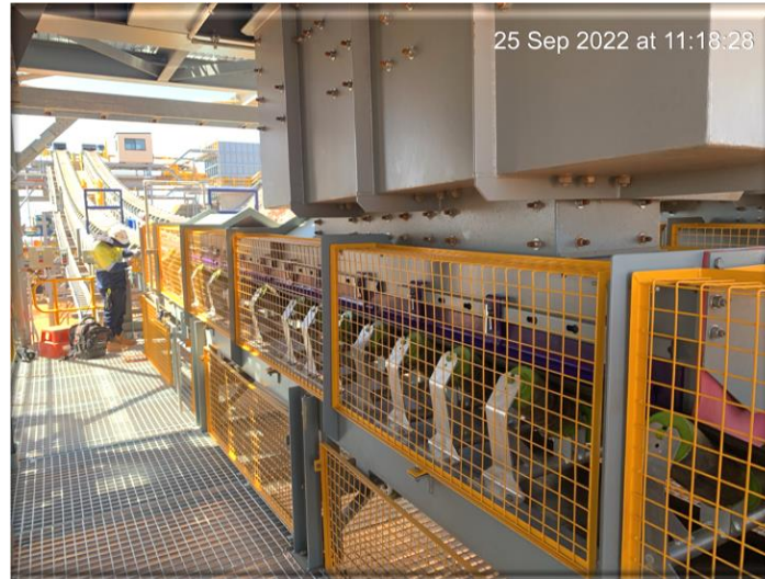
Screen section conveyor guarding
