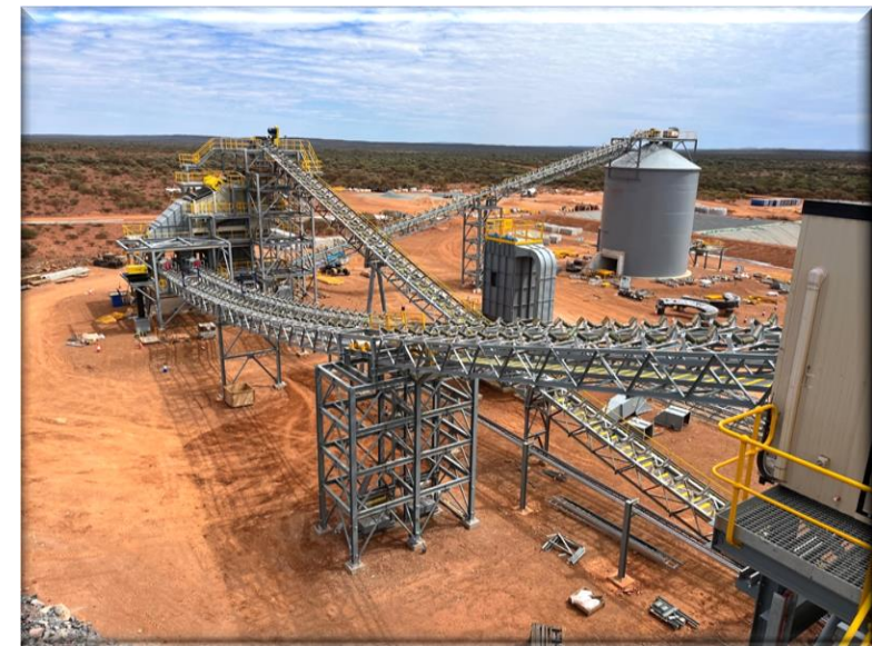
Plant screening & ore bin
