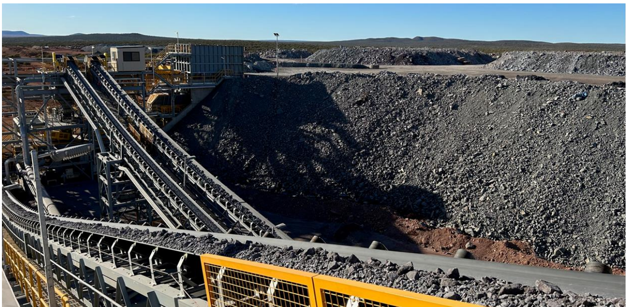
Figure 1 – Abra crushing circuit operating with ROM stocks in background (photo 3 May)
