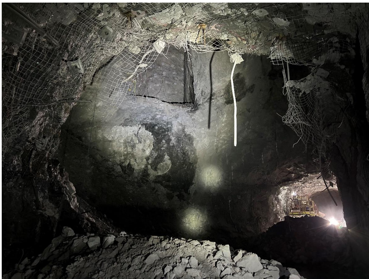
Figure 11 – Picture showing large underground stope at Abra on the 1280mRL level which will be paste filled in October after completion of mining (Photo 5 September 2023).
