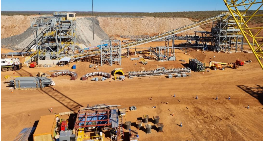
Figure 5: Photo showing construction progress crushing and screening circuit (July 2022).
