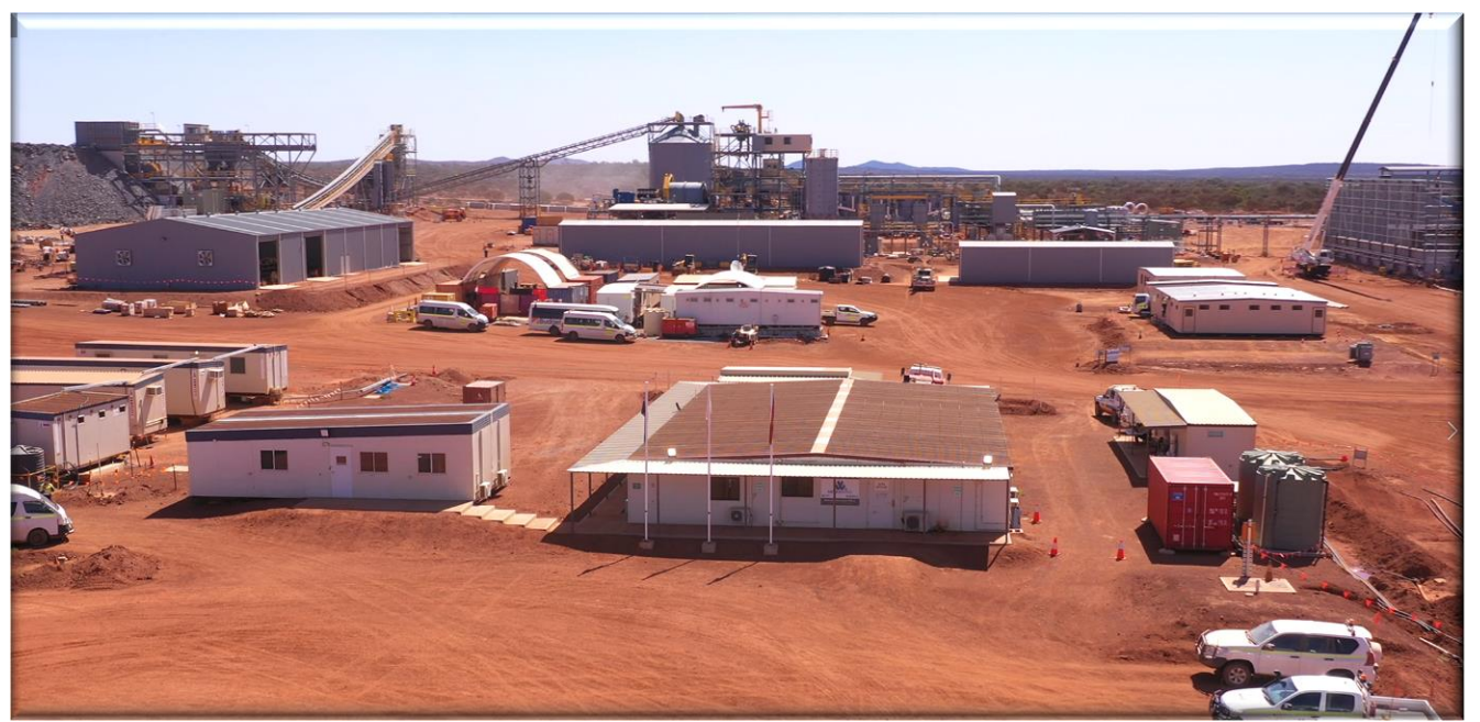
Mine Administration Building & Processing Plant
