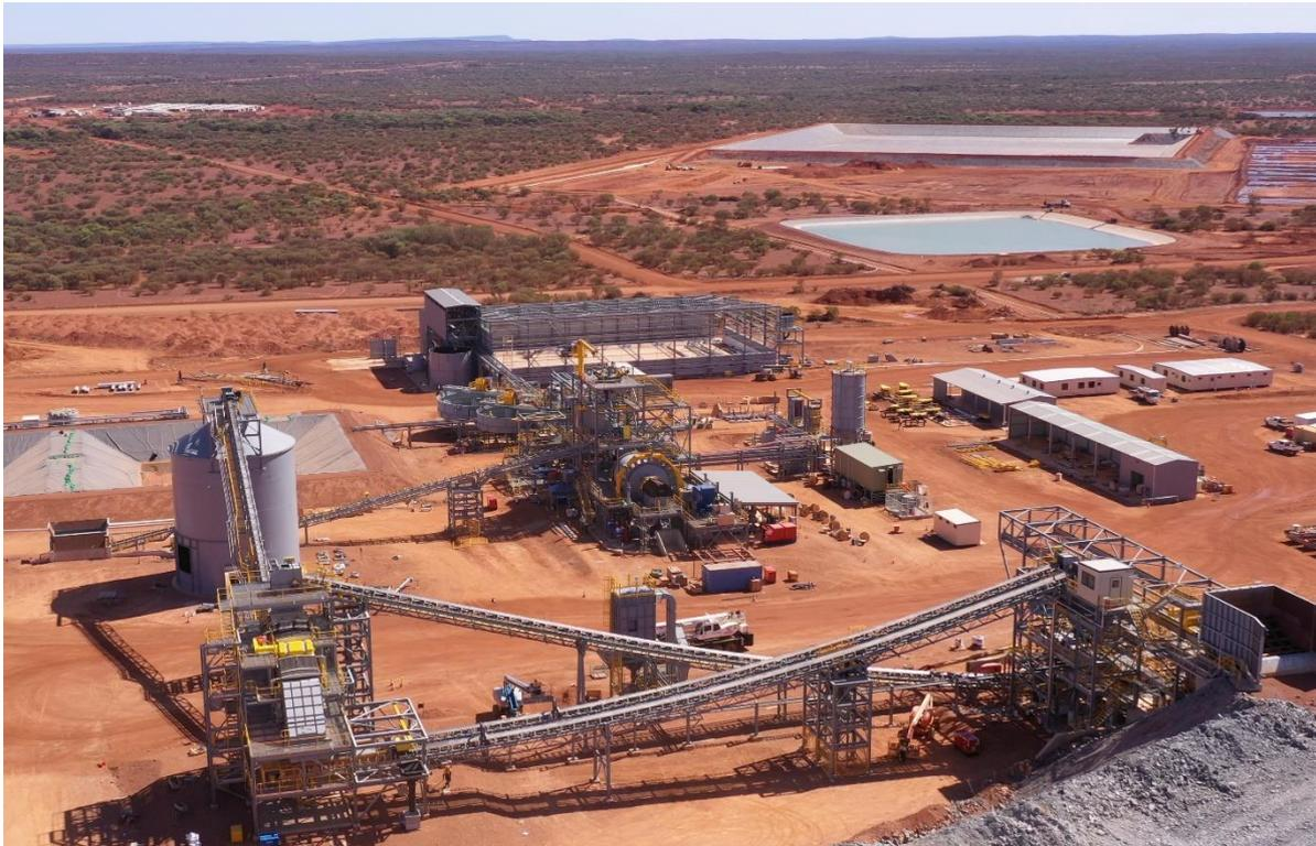
**Figure 1** – Processing plant with completed TSF and village in background (Photo 14 October).
