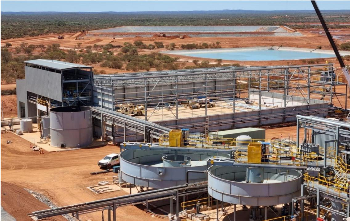
**Figure 7** – Abra Concentrate and tailings thickeners in front of filtering and storage section with completed TSF in the background (Photo 14 October).
