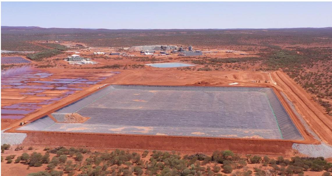
**Figure 8** – Completed TSF in the foreground with processing plant and box-cut in the background (Photo 14 October).
