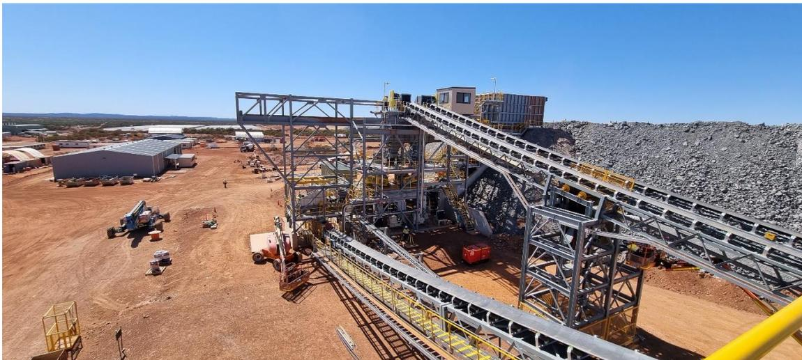
**Figure 6** – Abra crushing and screening area to commence dry commissioning in October. Site stores and plant workshop building seen on the left (Photo 14 October).
